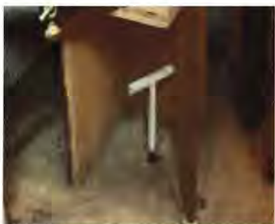
"T" handle used to operate stop&drain valve
