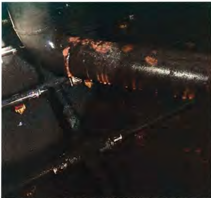
top wash (small with heads) and backwash (pitted) piping in Filter #1
